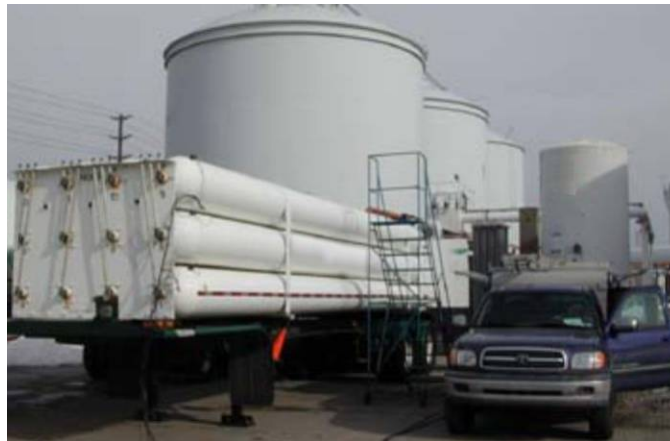
Figure 1. A typical steel tube trailer for transportation of fuel gases
